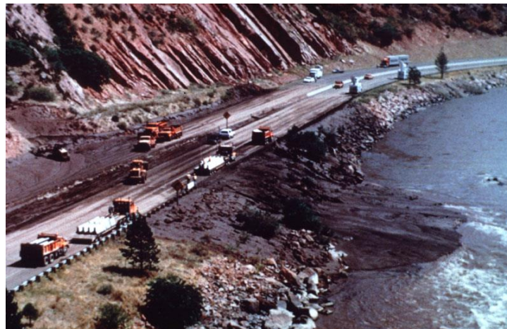
Landslide from fire damage in CO 74
