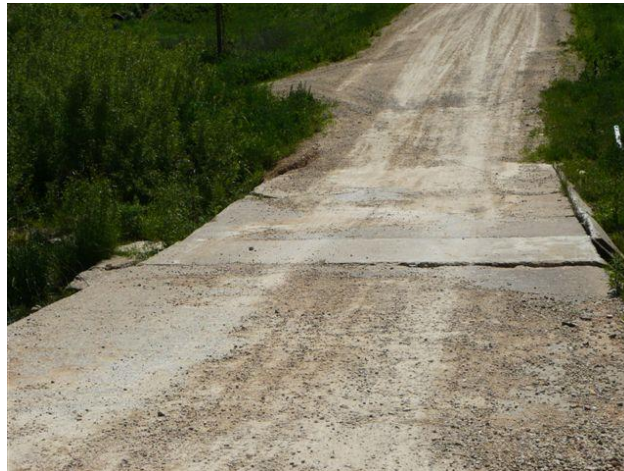
Richland County road with erosion due to overtopping of flood waters. 2009
