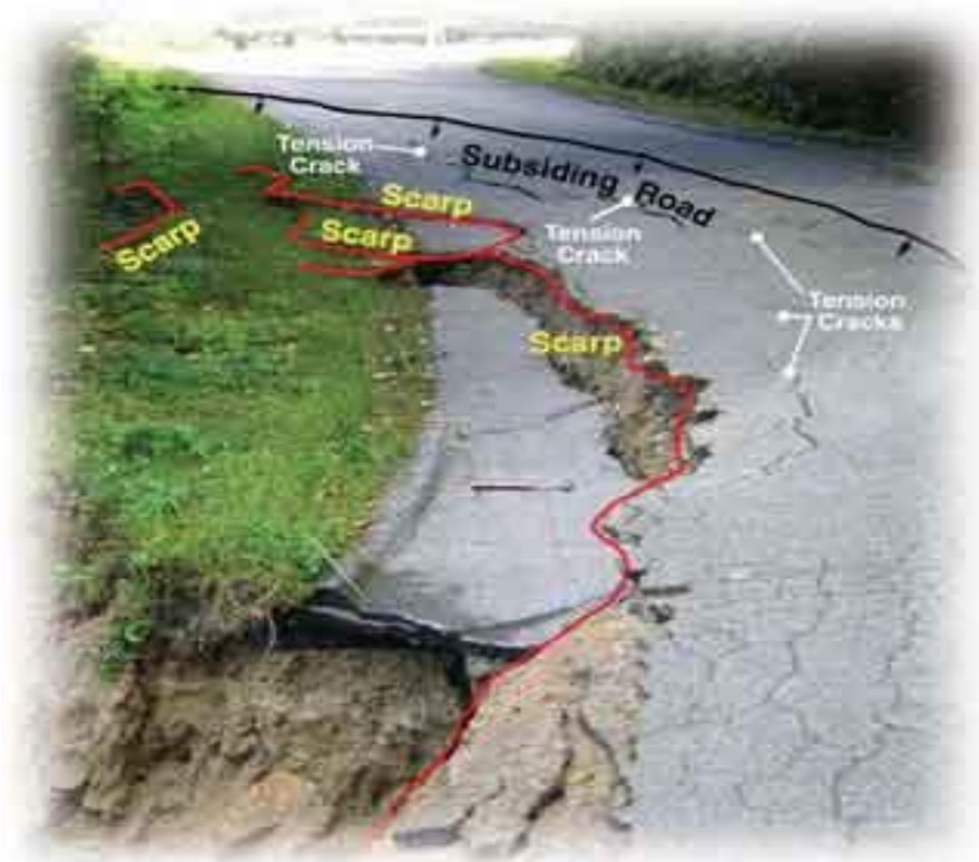
This picture shows landslide damage to a roadbed similar to that found in flash flood events in Richland County. 73
